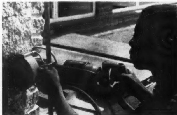
LEFT: The saw operated by a native is making a vertical test cut in a block of granite. The air hose is attached at the base of the handle; the water used as a coolant and to remove the cuttings flows through the tube alongside the air motor. RIGHT: Taking a horizontal cut. The supporting rod is not used, and one of the diamond saws has been removed.
